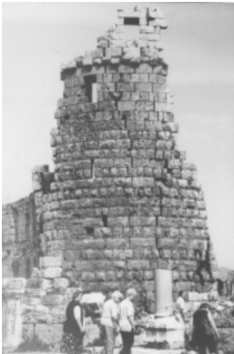
Fig. 3. Tower, Perge (Turkey).
