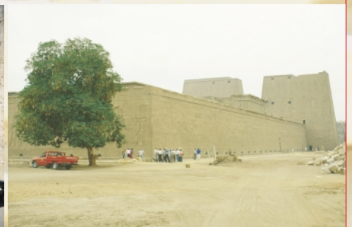
Outer wall and Grand Pylon
