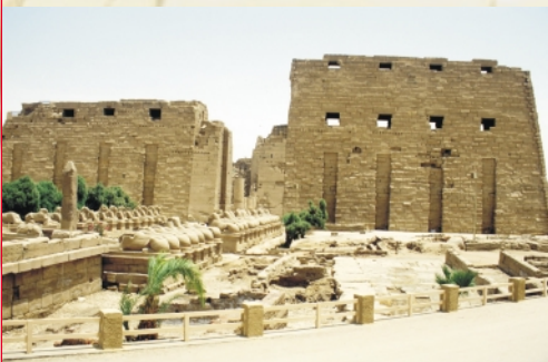
Avenue of the Sphinxes and 1 st Pylon
