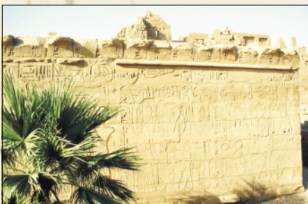
Karnak Temple, Ramesses III Temple, SSW - facade
