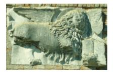
Weathering form: **Break out due to non-recognizable cause (oO)**
