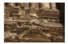
Weathering form: **Break out due to natural cause (nO)**
