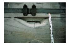
Weathering form: **Break out due to constructional cause (bO)**
