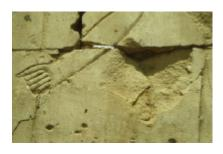
Weathering form: Break out due to non-recognizable cause (oO)
