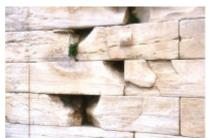
Weathering form: Break out due to non-recognizable cause (oO)
