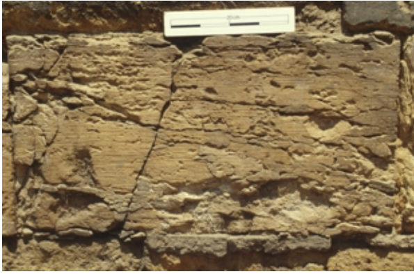
Fig. 15. Weathering forms ‘relief (R)’, ‘break out (O)’, ‘crumbly disintegration (P)’ and fissures (L)’. Image width appr. 70 cm.
