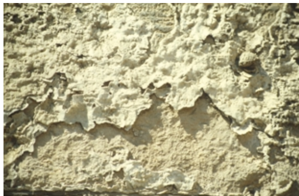
Fig. 14. Weathering forms 'back weathering (W)', 'crust (C)', 'detachment of crusts with stone material (K)' and 'granular disintegration (G)'. Image width appr. 30 cm.
