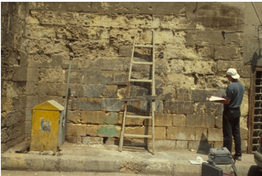
Fig. 16. El-Merdani Mosque - lower part of the SE-façade.
