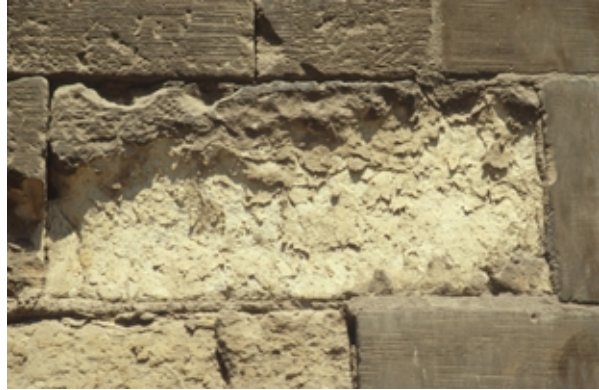
Fig. 12. Weathering forms 'back weathering (W)', 'crust (C)' and 'flaking (F)'. Image width appr. 70 cm.
