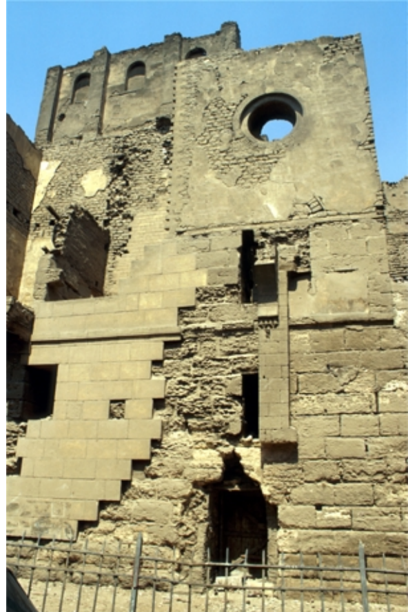
Fig. 8. Stone replacement. Hospital of Sultan Al-Mansur Qalawun.
