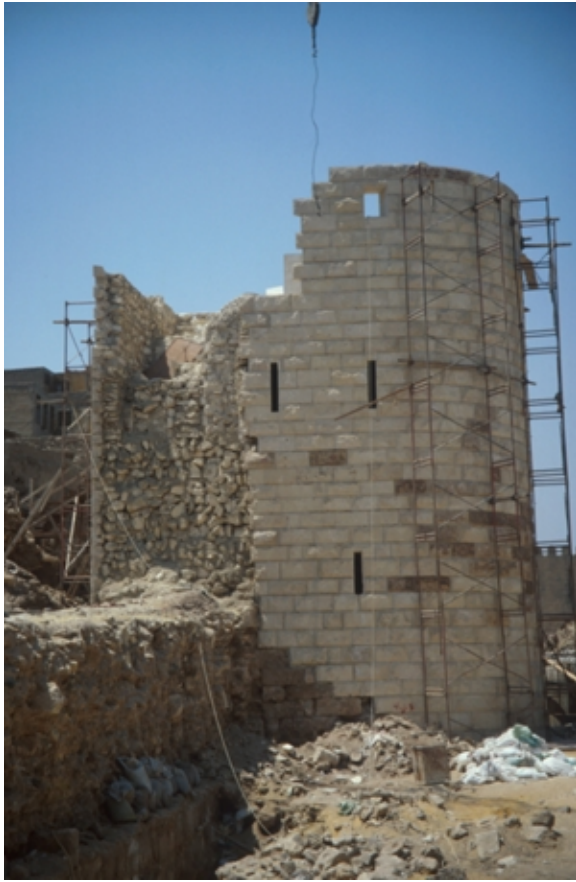
Fig. 9. Restoration works. Northern wall of Cairo.
